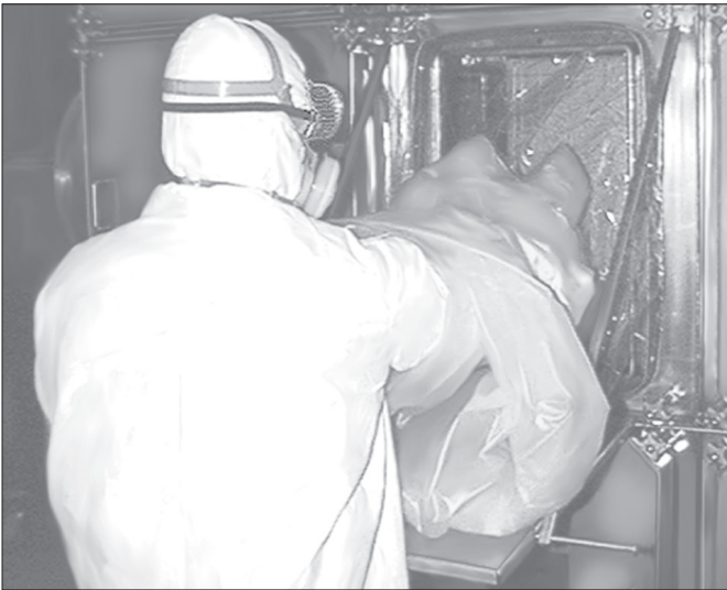
Place hands and arms in filter removal glove sleeves.
