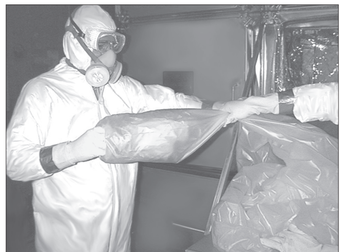
Grip bag while turning glove sleeve inside out.
