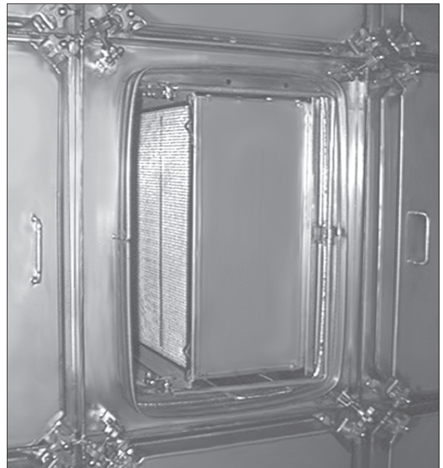
Locking mechanism latched with filters installed.
