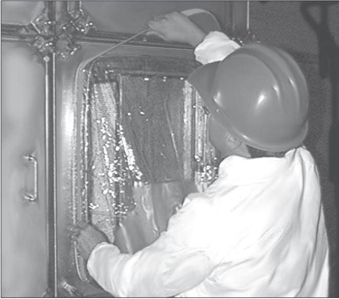
Locate D-Ring on strap at top of bag-in/bag-out ring before tightening.
