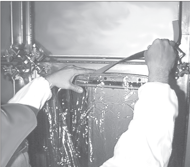
Pull strap until it is tight around the bag-in/bag-out ring. Press Velcro together. Secure excess strap so it will not interfere with the door seal.
