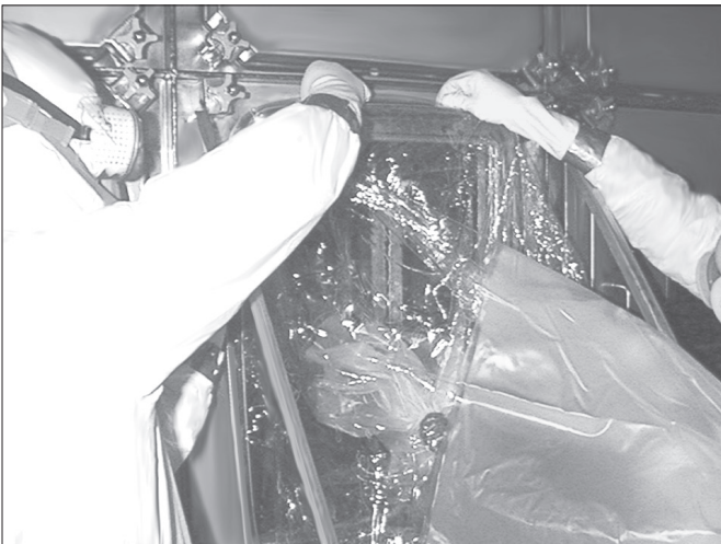
Place new bag on ring over the old bag stub.
