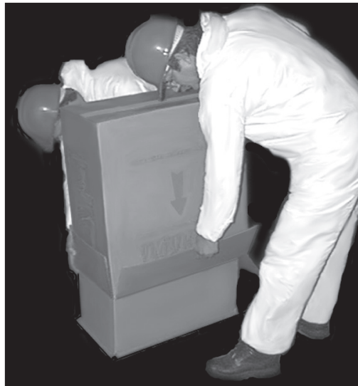
Rest filter on floor while removing carton.
