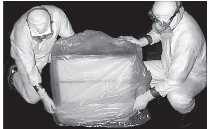
Pull remainder of bag down over filter.
