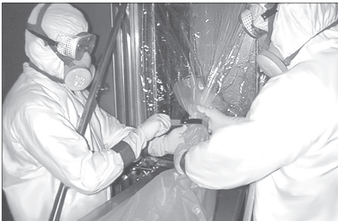
Cinching strap installation.
