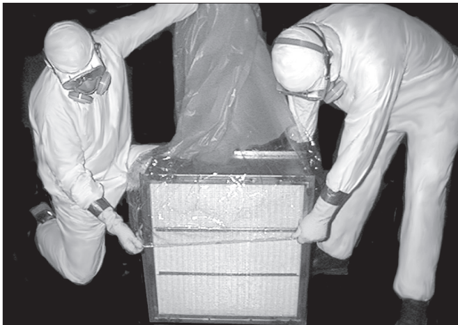
Carefully pull shock cord of bag to bottom of filter.
