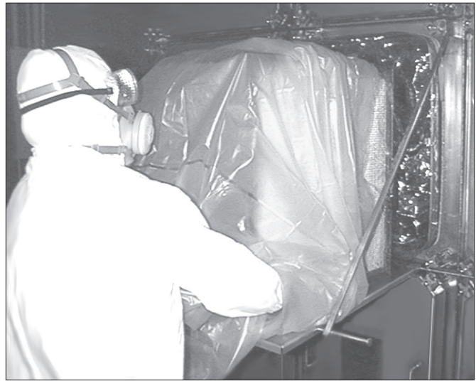
Place filter on sturdy table, stand, shelf, or floor. Remove arms from bag, leaving glove sleeves inside.
