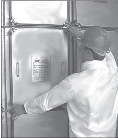
Remove aluminum knobs.
