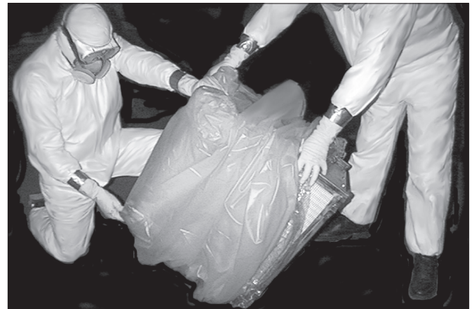
Pull bag down until filter is at back of bag.
