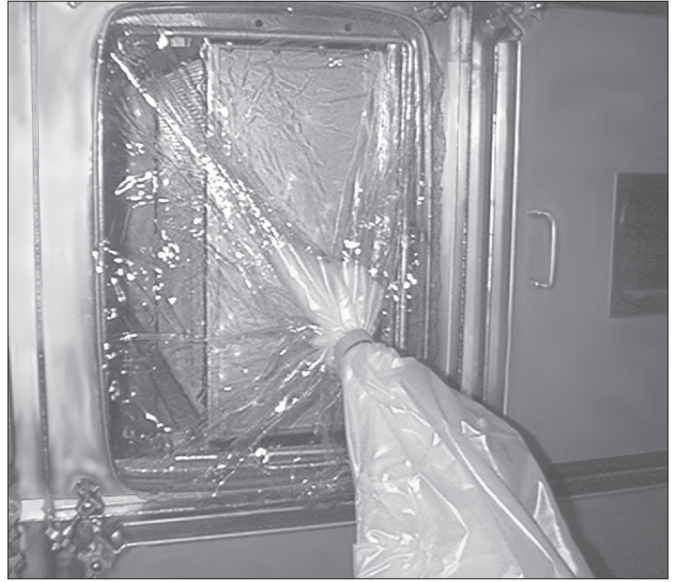
The nylon cinching strap helps minimize the possibility of the bag being drawn into the housing during operation.
