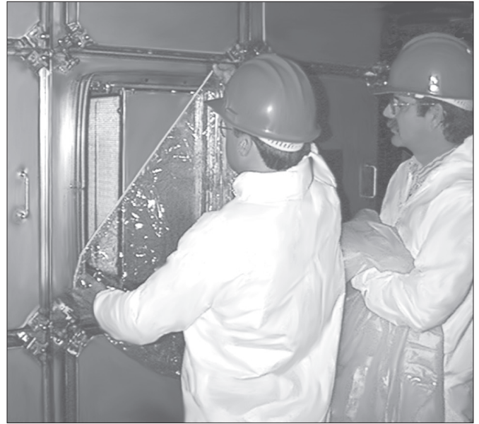
It is easier to work bag from bottom to top of bag-in/bag-out ring. Locate seam of bag at top of ring, so gloves in bag are in the correct position.
