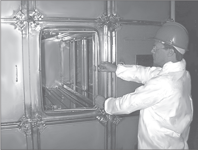
Release filter locking arm from handle latch.
