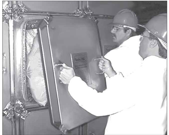
Filter access door tightening sequence.
