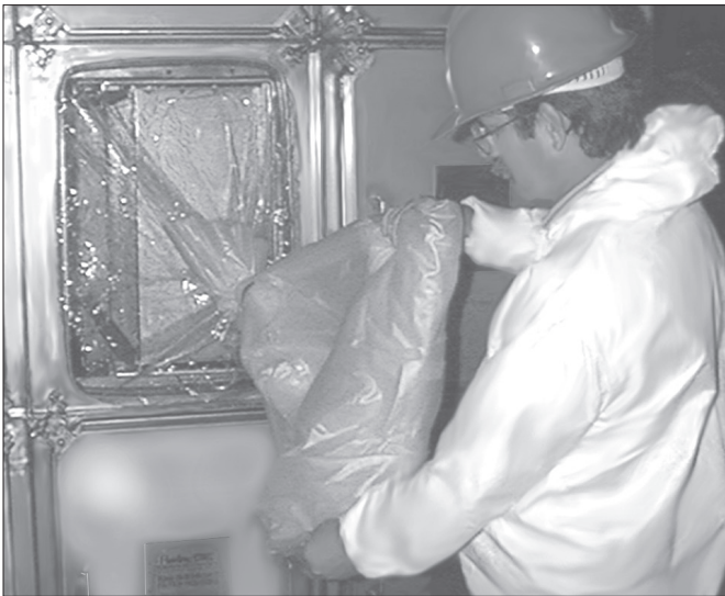
Filter access door tightening sequence.
