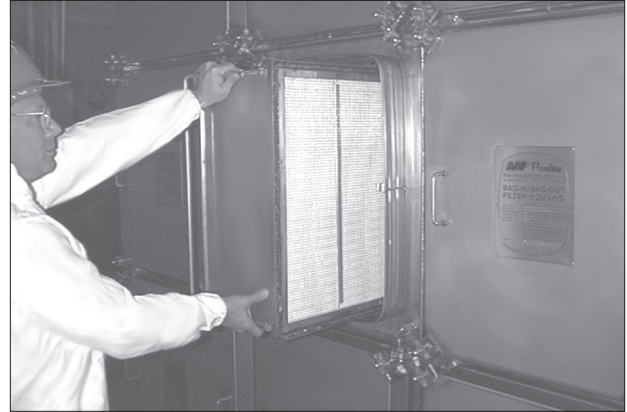
Install HEPA filters with pleats in vertical position.
