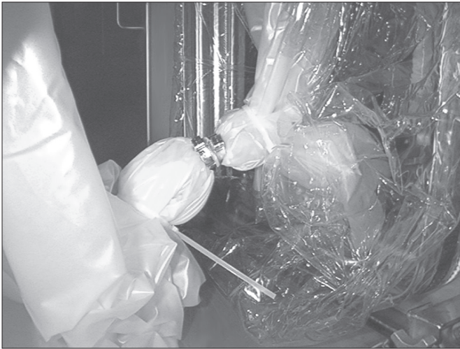
Using the AAF Flanders optional Banding Kit, cinch with metal bands.
