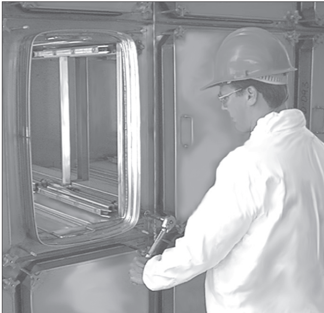
BG-Series Gasket Seal Housing inside view showing the filter locking mechanism. Note the exterior drive bolts and spring-loaded mechanism.
