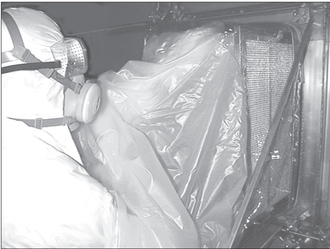
Slowly and carefully remove filter from housing; hold filter at top and bottom of frame.
