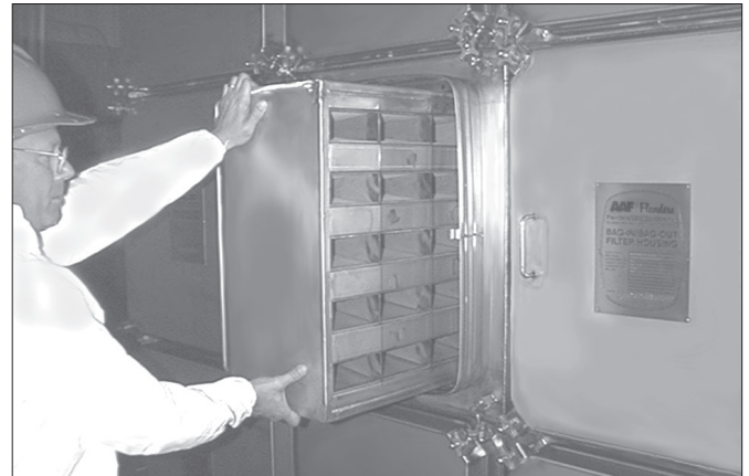
Install adsorbers with beds in horizontal position.
