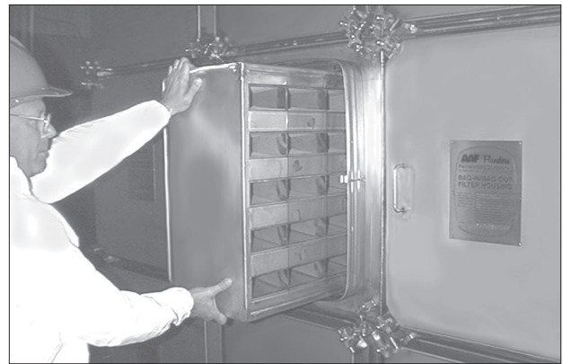
Install adsorbers with beds in horizontal position.
